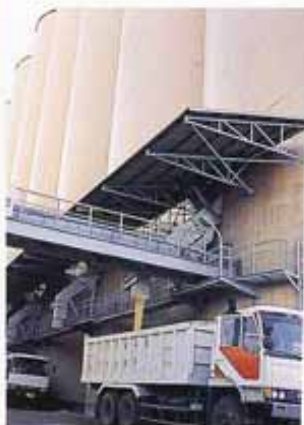
트럭적상차구 / Truck Load-Out Spout
